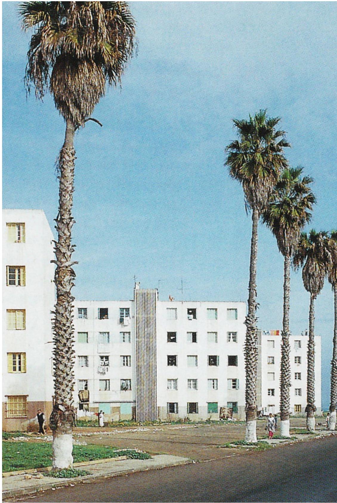
J. H. Laure: housing complex, El Hank (1953) Photograph taken by Jean-Louis Cohen in 1991
