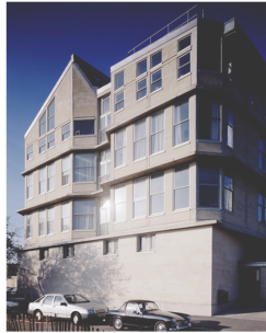
School of Architecture & Building Engineering Alison & Peter Smithson
