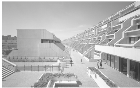
Alexandra Road Estate Neave Brown
